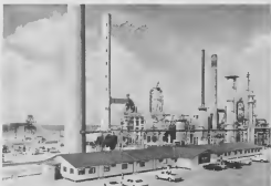
View of new HDS-II facilities built on reclaimed land.
